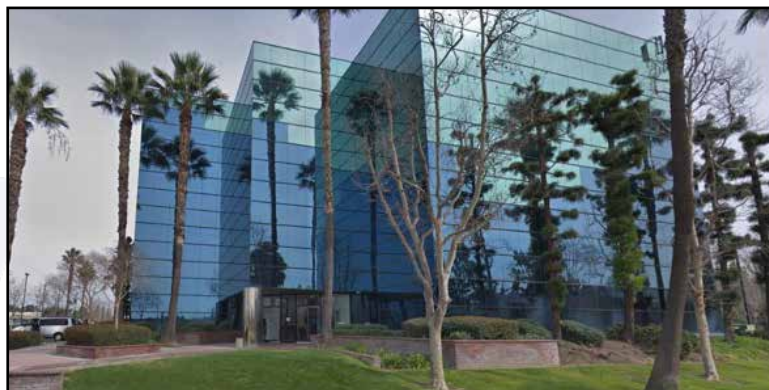
2015 – Current - 268 West Hospitality Lane Auditor-Controller/Treasurer/Tax Collector Office of Central Collections This building now serves as the headquarters for all taxpayers and staff in one location, including the functions of the Auditor-Controller/Treasurer/Tax Collector.
